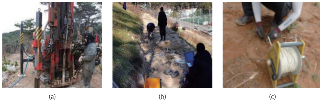
그림 2. Geophysical prospecting (a) Boring (b) Seismic survey (c) Groundwater level measurement
